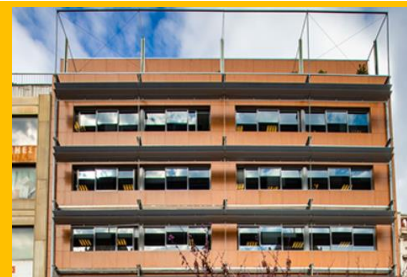
67, Aioulou Str, Athens Eight-storey building, 3.022 sqm
